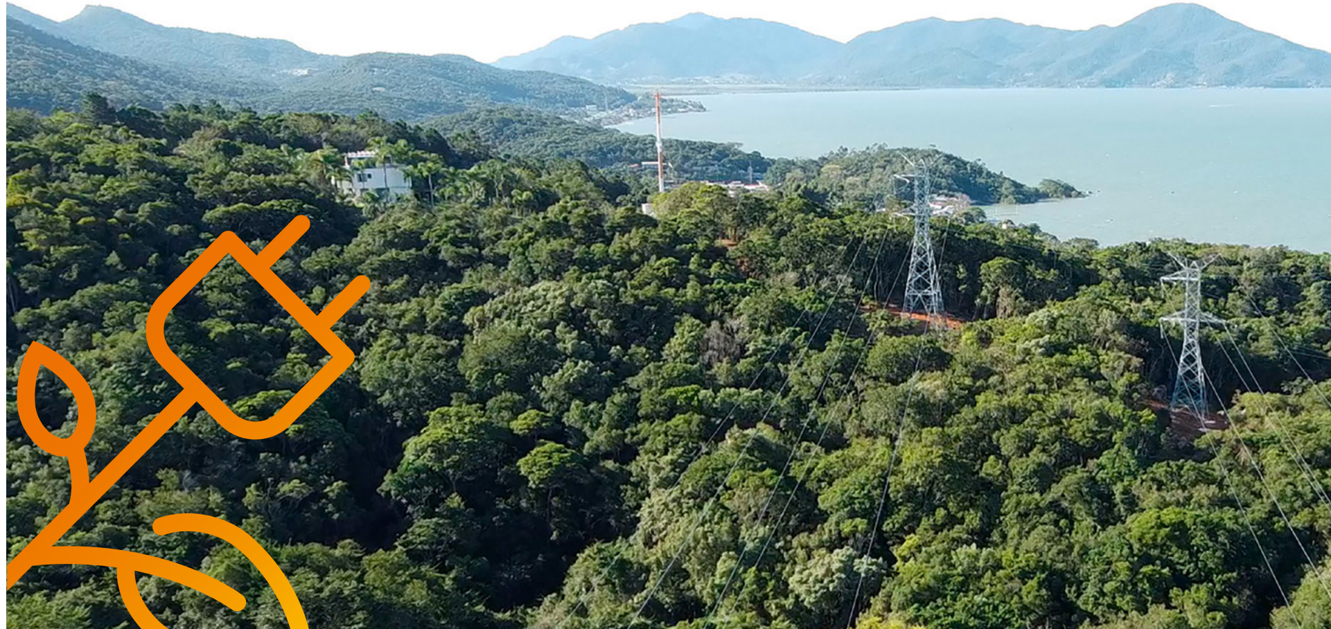
• Biguaçu Electrical Interconnection (SC)
